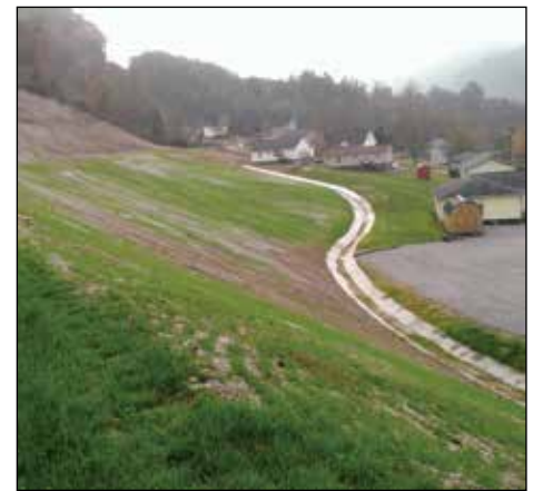
OPPOSITE PAGE: Excavation began on the steep hillside where 97,365 cubic yards of slide material were removed to prevent further damage to the homes below. Photo by Ben Enzweiler, AML. THIS PAGE (left to right): post-reclamation fill area beside the Harlan County Detention Center; Yocum permit site near the Evarts High School after reclamation; excavation is complete and drainage control measures route surface and groundwater away from the homes. Photos by Carl B. Hays
