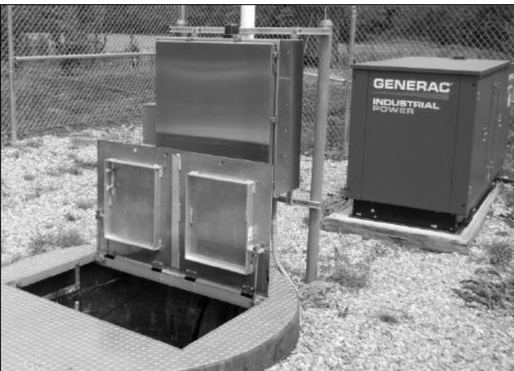
A new lift station on Lawrence Street in Livermore.
